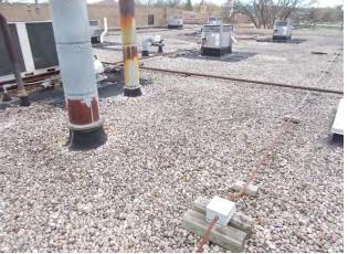
5. Ownership should consider replacement of the drains on Roof Areas 1 & 2 in conjunction with the roof replacement. These drains appear to be original and have been a source of leakage.
