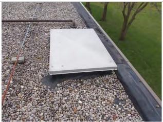
3. It is recommend that the adhered rubber walkway pads be replaced with 2' x 2' x 2" interlocking rubber pavers (to and around all serviceable equipment) to ensure adequate protection of the roof membrane in high traffic areas. These pavers should also be added to the east perimeter of Roof Area 3, where fire department personnel reportedly access the roof edge during training exercises. Currently a wood platform is constructed.
