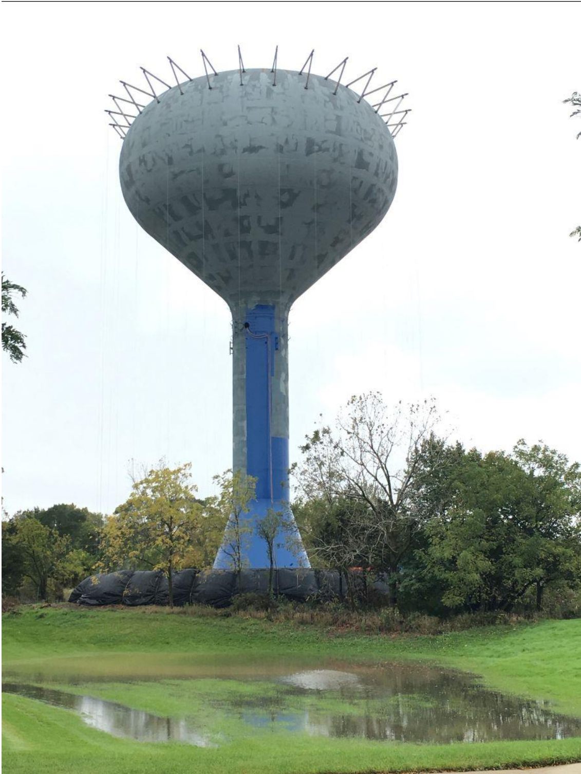
The Knowles Road Water Tower is currently being painted internally and externally to protect against rust and other damages
