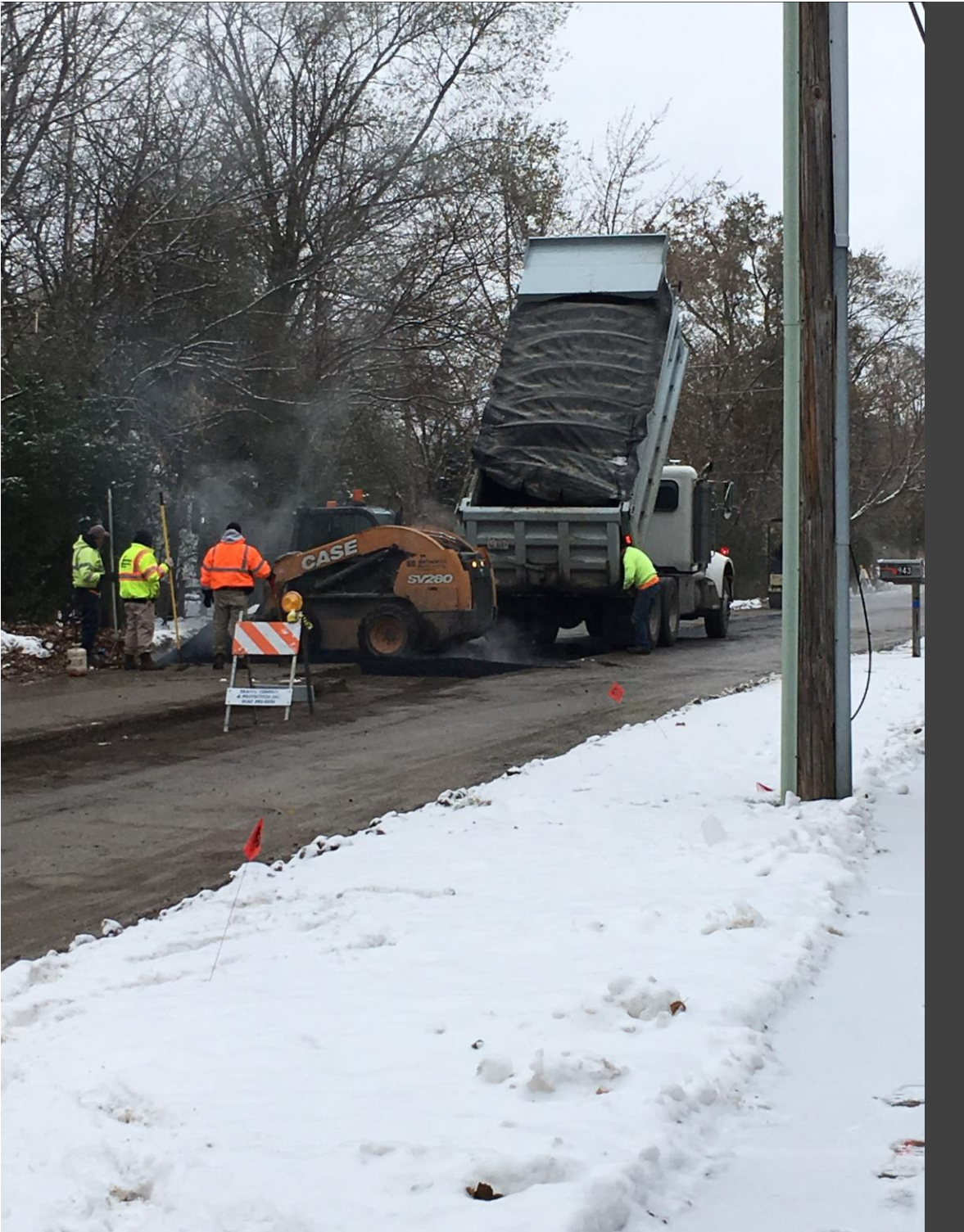
Lenny Hoffman Excavating completed the water main project along Delany Road on November 22nd and it is now open to traffic.
