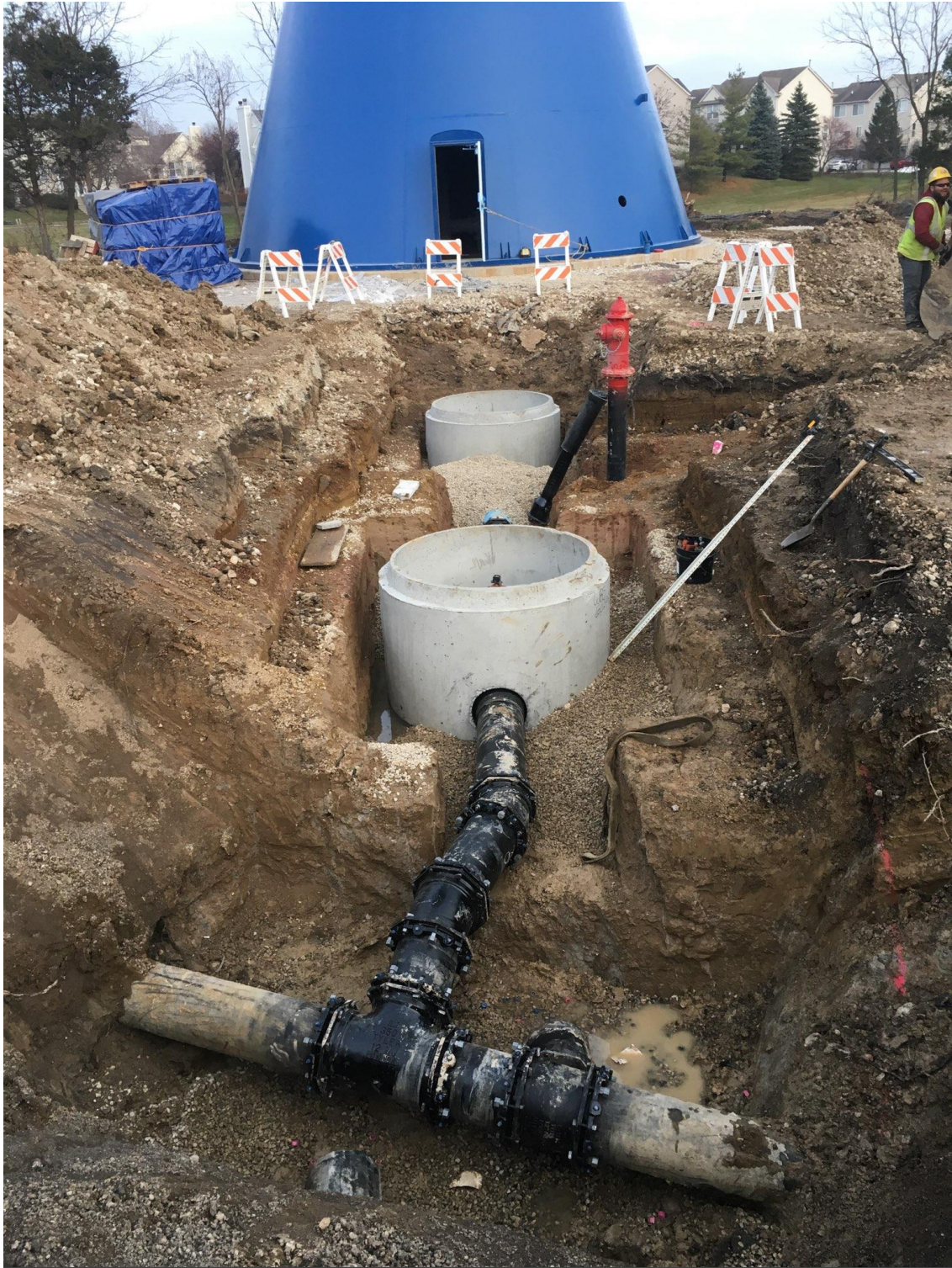
Due to the weather restricting the painting of the water tower, contractors work to install the water main pipe connecting the tower to the existing main.
