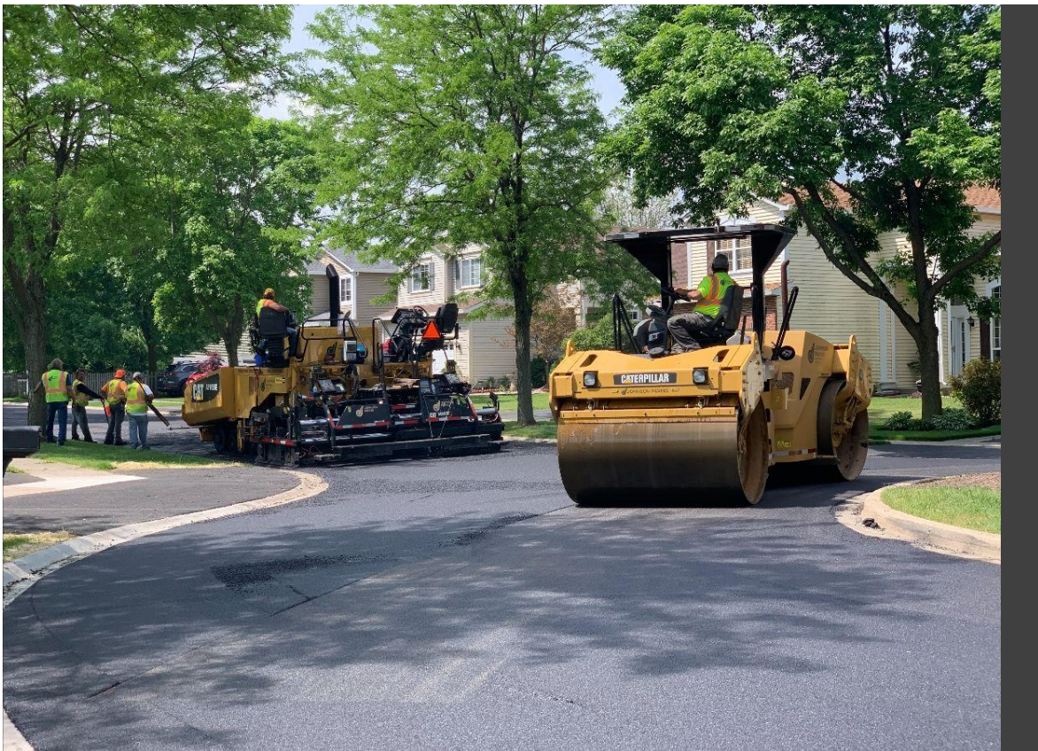
Crews completing paving of a roadway.
