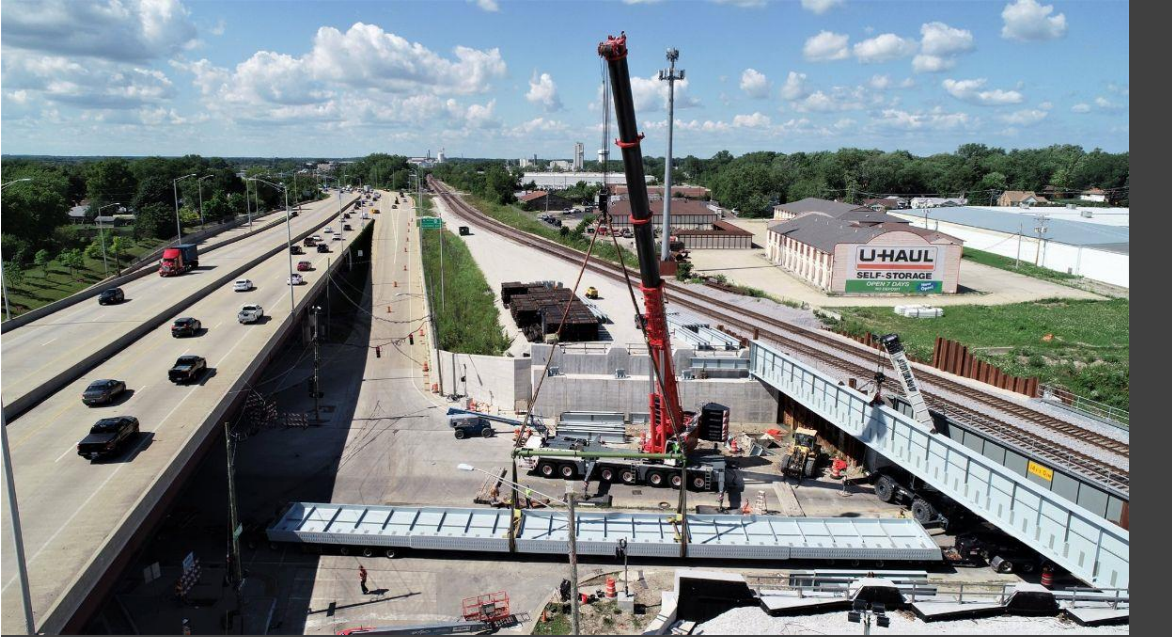
Photo courtesy of T.Y. Linn, IDOT's construction project engineer for the Route 41 / Grand Avenue Bridge Widening Project
