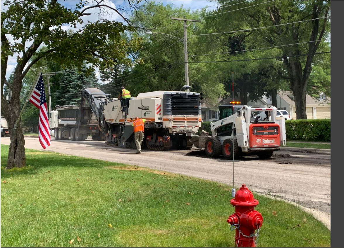
Crews completing paving of a roadway.
