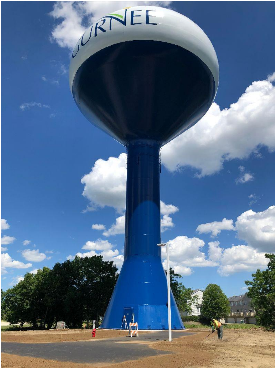
Knowles Road Water Tower #5
