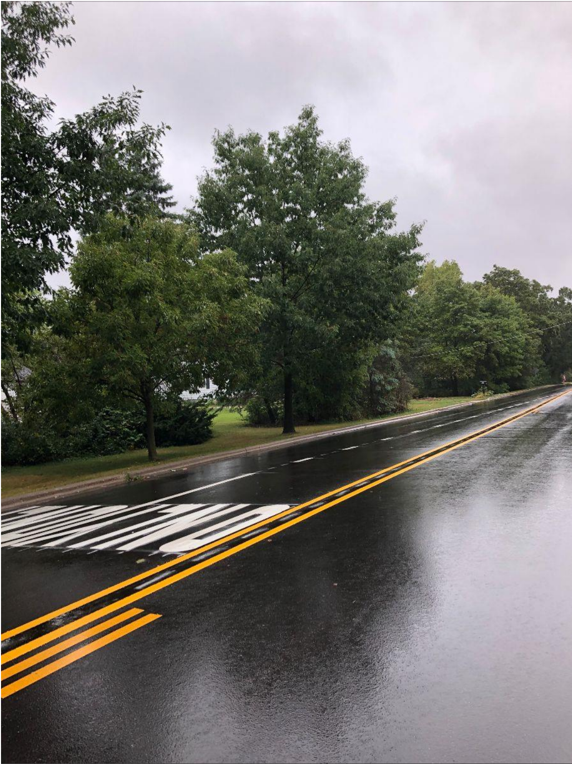
A newly resurfaced and painted roadway as part of the 2020 construction program.
