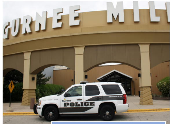
Gurnee Mills which houses a Police Substation
