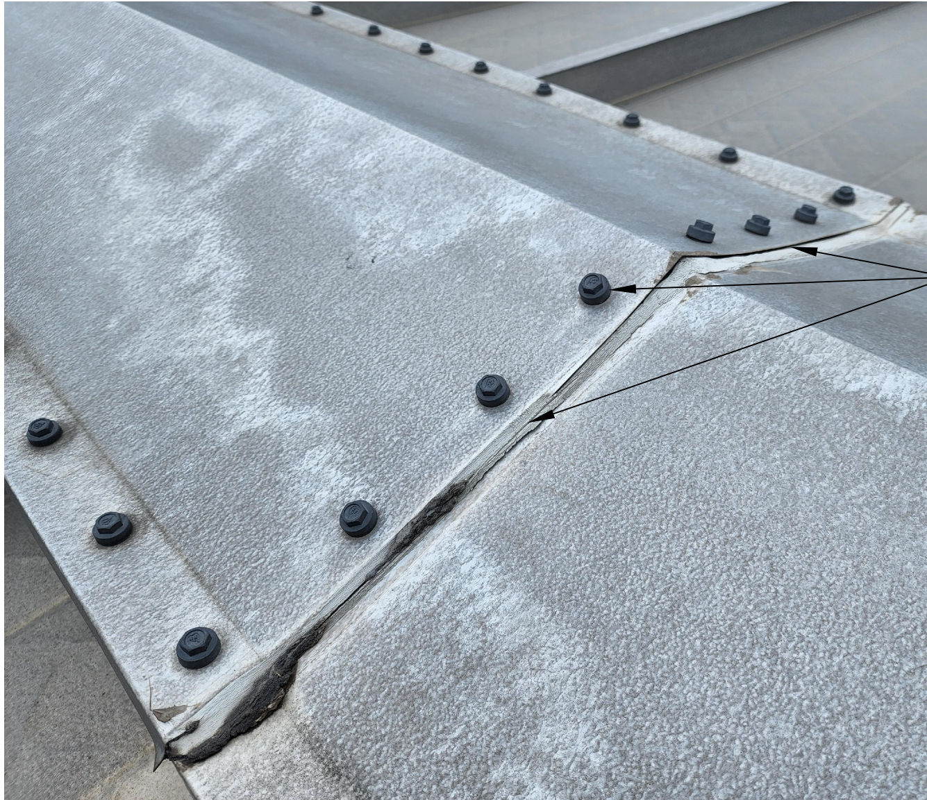
8 RIDGE CAP SEAMS SCALE: NTS
