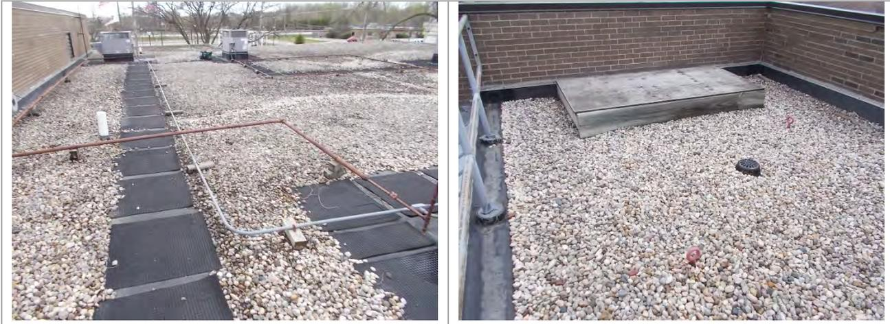
4. The roof replacement should include replacement of the deteriorated wood pipe supports where pipes run across the roof surface. (this would be required if additional insulation is installed)
